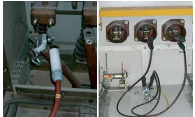
➤ single phased connection, not involved phases grounded
