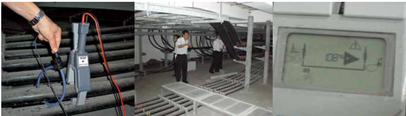
➤ Field Application of Cable Identification
